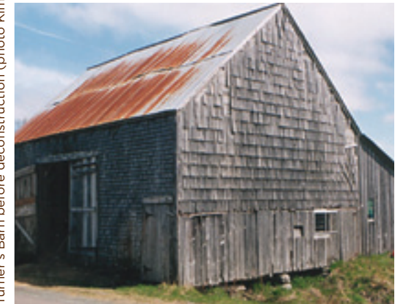
Turner's Barn before deconstruction (photo: Kim Aaboe)
