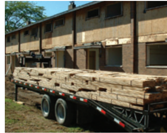
Deconstructing PMQs (photo: Joseph Colp, Defence Construction Canada)
