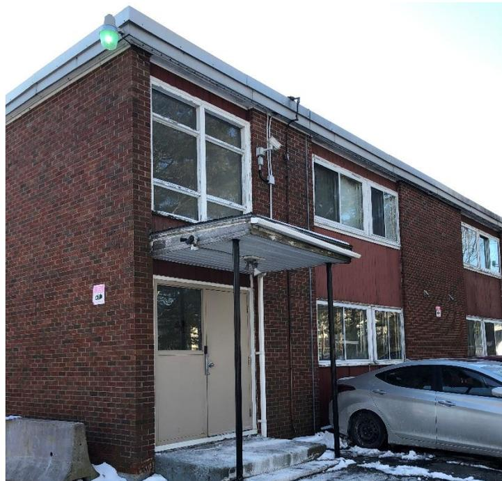
Figure 5.1 Existing Brick & Wood Panel Enclosure
