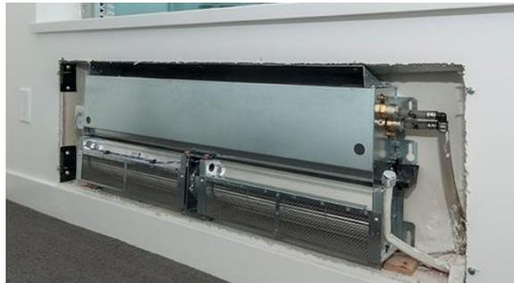
*Figure 8.2 - Example of a Perimeter Fan Coil Unit Replacing a Radiator*
