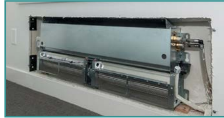
Example of a Perimeter Fan Coil Unit Replacing a Radiator
